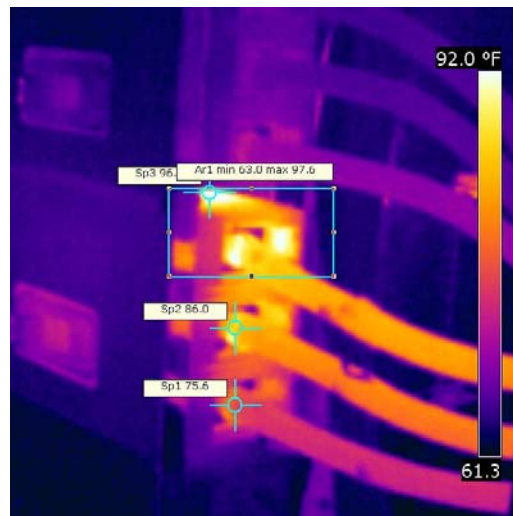
Fig 5 – Temperature Differences between Three Sockets
